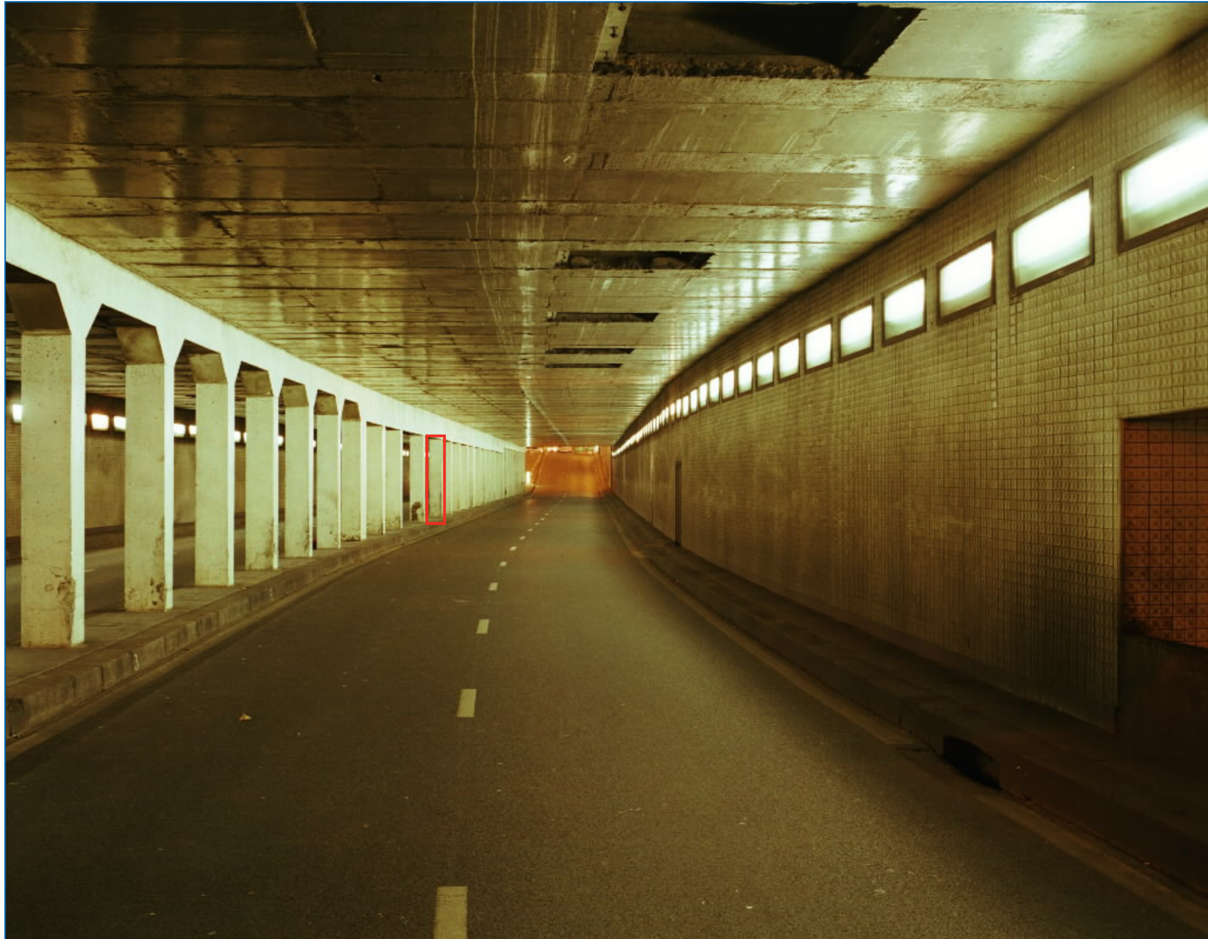
Alma underpass, 13th pillar highlighted
